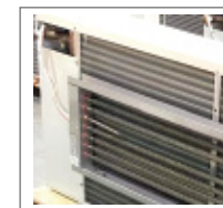
External Re-heat Coil
